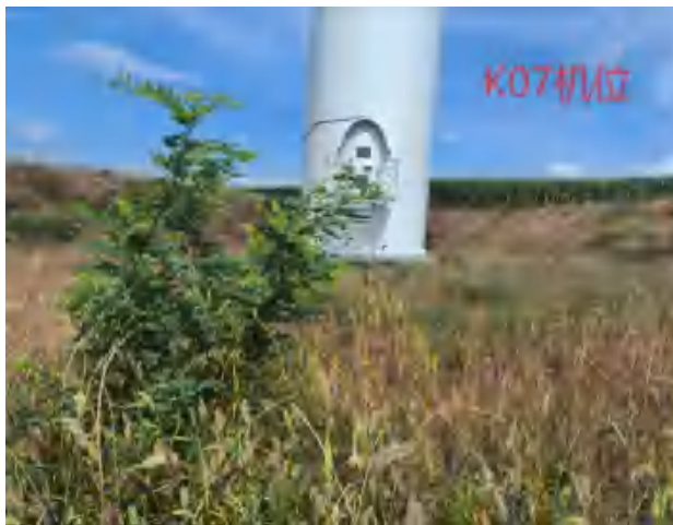
K07 风机吊装平台生态恢复
